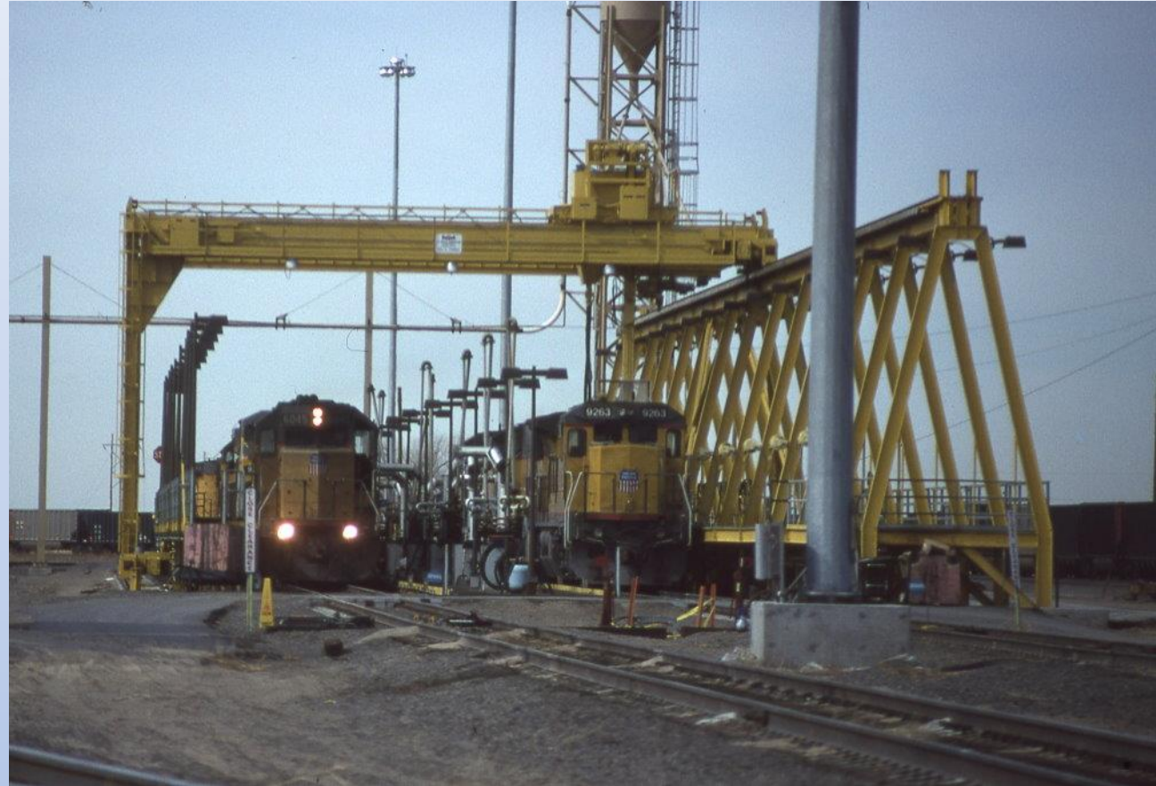
West Service Track at UP Bailey Yard, N Platte, NE
