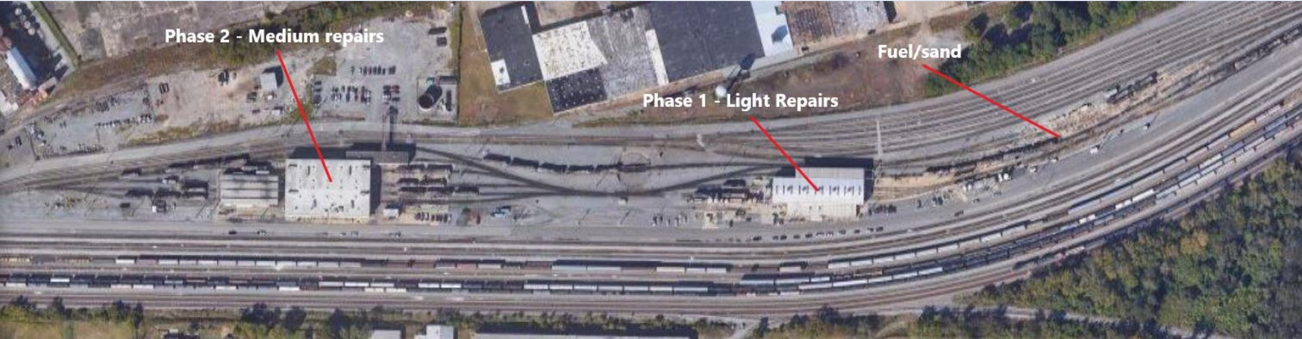
Locomotive Shops, MP N Little Rock Yard
